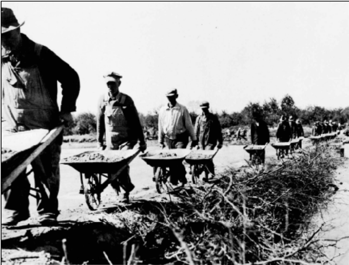
Works Progress Administration (WPA) men work on an Arkansas River flood control project May 17, 1939.
